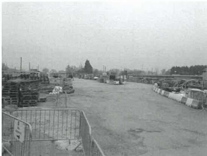
Site looking south from northern boundary.
