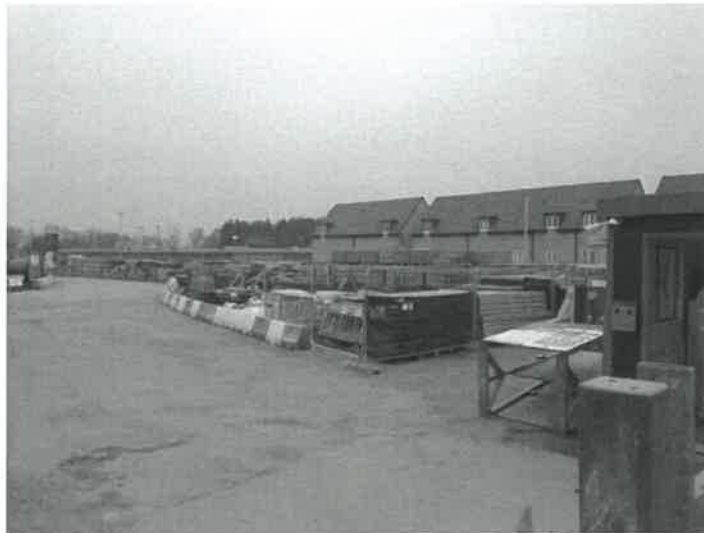
Site looking south west from northern boundary.
