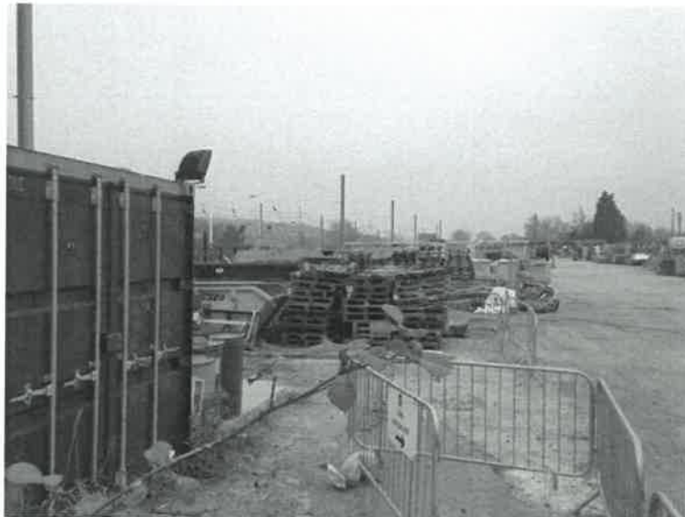
Site looking south east from northern boundary.
